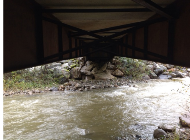
Right Bank Abutment when facing downstream
