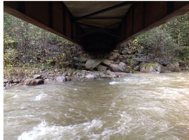
Left Bank Abutment when facing downstream
